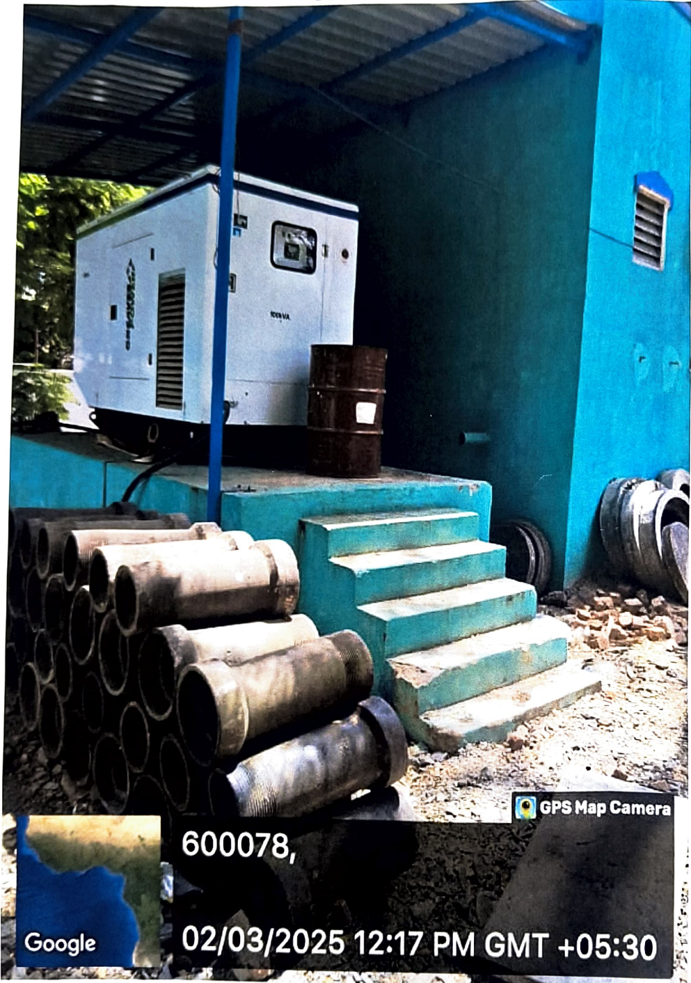
K.K.Nagar "A" Newly constructed at Alagirisamy salai
